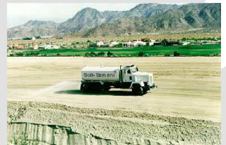
Soil-Sement® applied to a construction site ...
