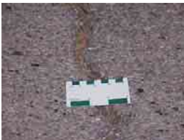
Figure 3b Moderate Transverse Cracking
