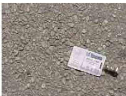
Figure 1a Slight Raveling
