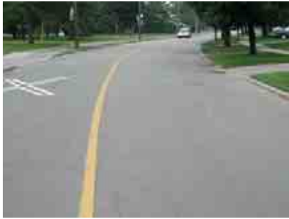
Figure 4a Slight Alligator Cracking
