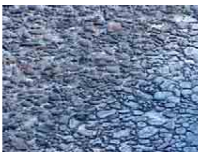
Figure 1b Moderate Raveling
