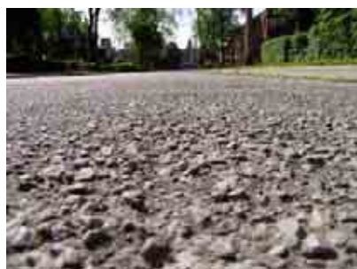
Figure 1c Severe Raveling
