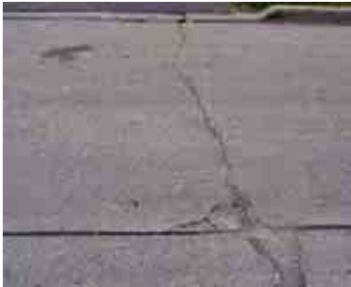
Figure 3a Slight Transverse Cracking
