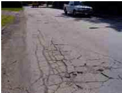
Figure 4c Severe Alligator Cracking
