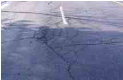
Figure 4b Moderate Alligator Cracking
