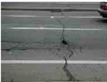
Figure 3c Severe Transverse Cracking
