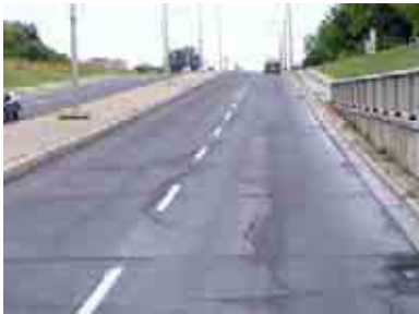
Figure 2.b Moderate Longitudinal Cracking
