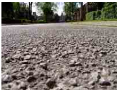
Figure 1c Severe Raveling
