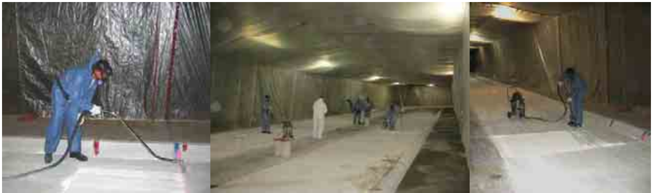
Figure 12: Vacuuming of Residue Material
