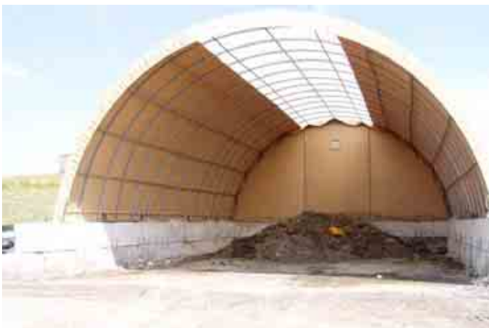
Figure 9: Enclosed Street Sweeping Pit
