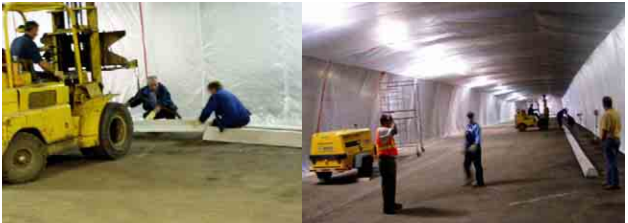
Figure 5: Construction of Enclosure and Installation of Portable Curbs
