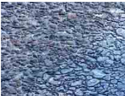
Figure 1b Moderate Raveling
